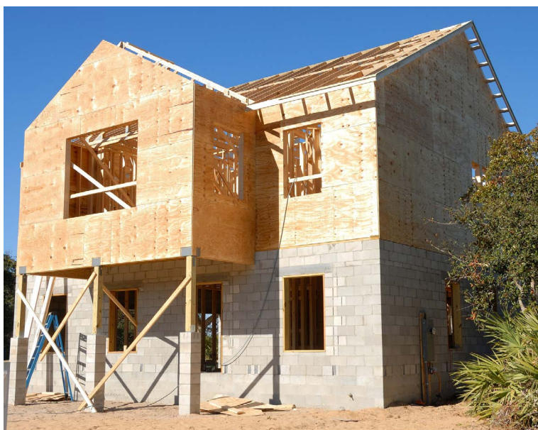
House under construction © paulbr75, pixabay, 2016
